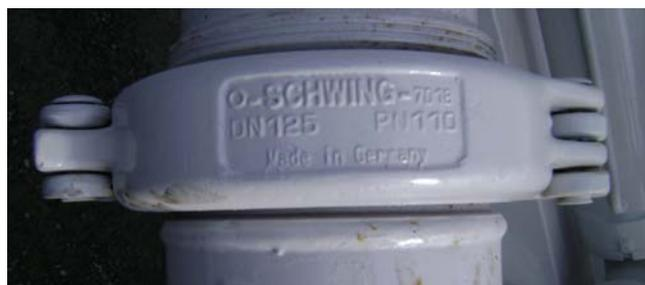
**Photograph 4:** An example of acceptable marking on pipe clamps.
